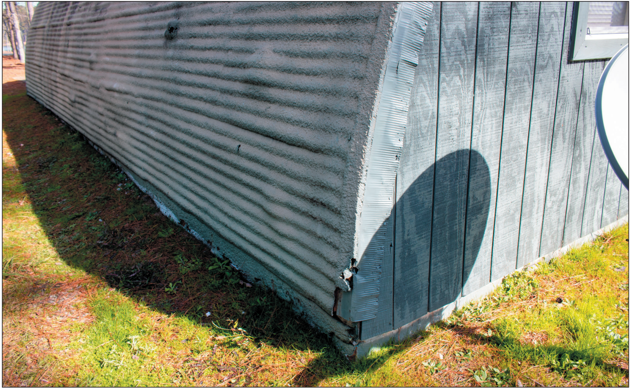
Figure 8. Edgewood Hut, Corner Detail Showing Foundation and Spray Foam Covering
