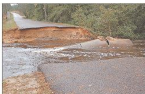
No. 2 - An overflowing McTier Creek washed away this part of Cumbee Trail Road in the Ridge Spring-Monetta area after heavy rains in October.
