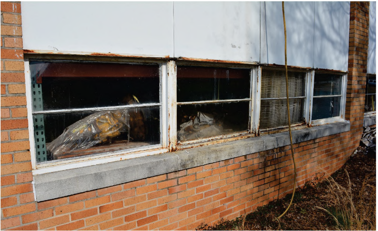
Figure 13. Close-up showing the metal casement windows and covered glass blocks above.
