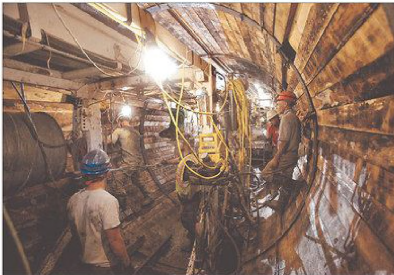
PHOTOGRAPH BY BRAD NITTEL/STAFF Construction workers with Triad-Midwest Mole install steel ribs and hardwood lagging on the outer wall of the 1,228-foot drainage tunnel under Market Street. The excavating process is complete and the next phase will be installing concrete walls.
