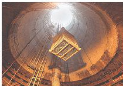
One of the ways construction workers gain entry to the Concord and Market streets drainage tunnels is by being lowered in a steel cage 140 feet below the ground.
