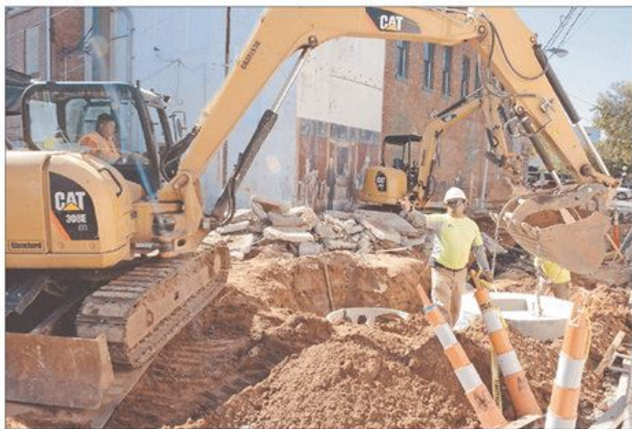
The Alley's renovation project, shown here in its Oct. 21 condition, is to include new water and sewer lines as well as burial of utility lines.
