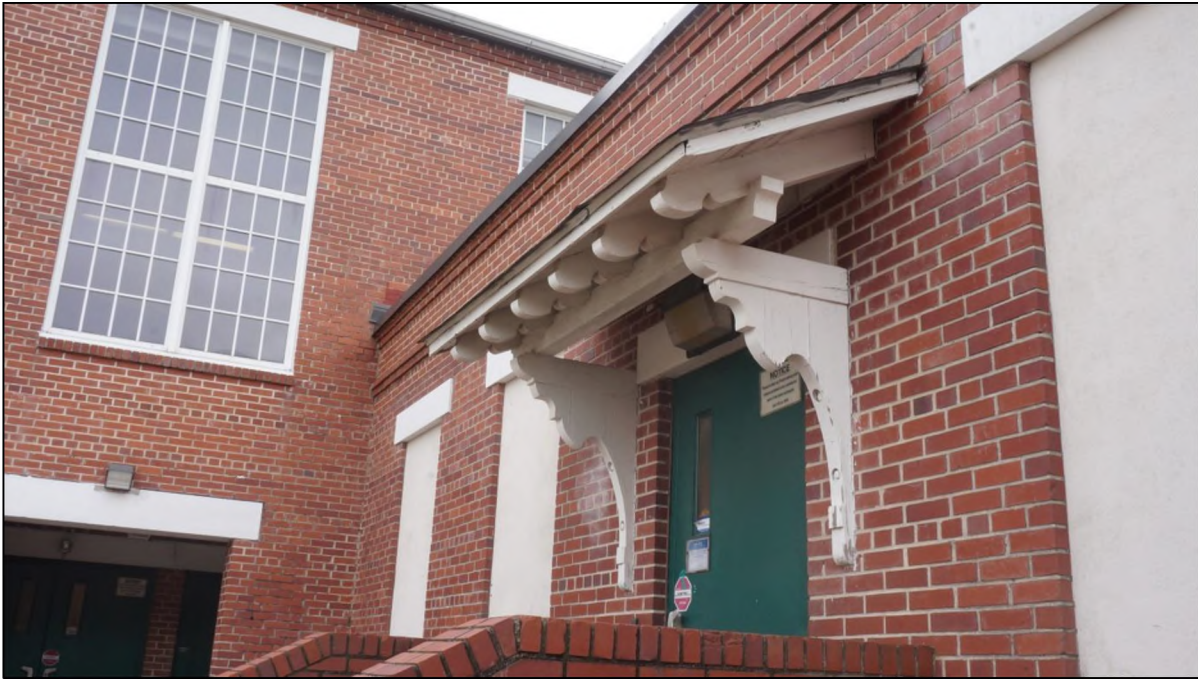
Figure 26. Decorative wood work supporting the shed roof above the stoop.
