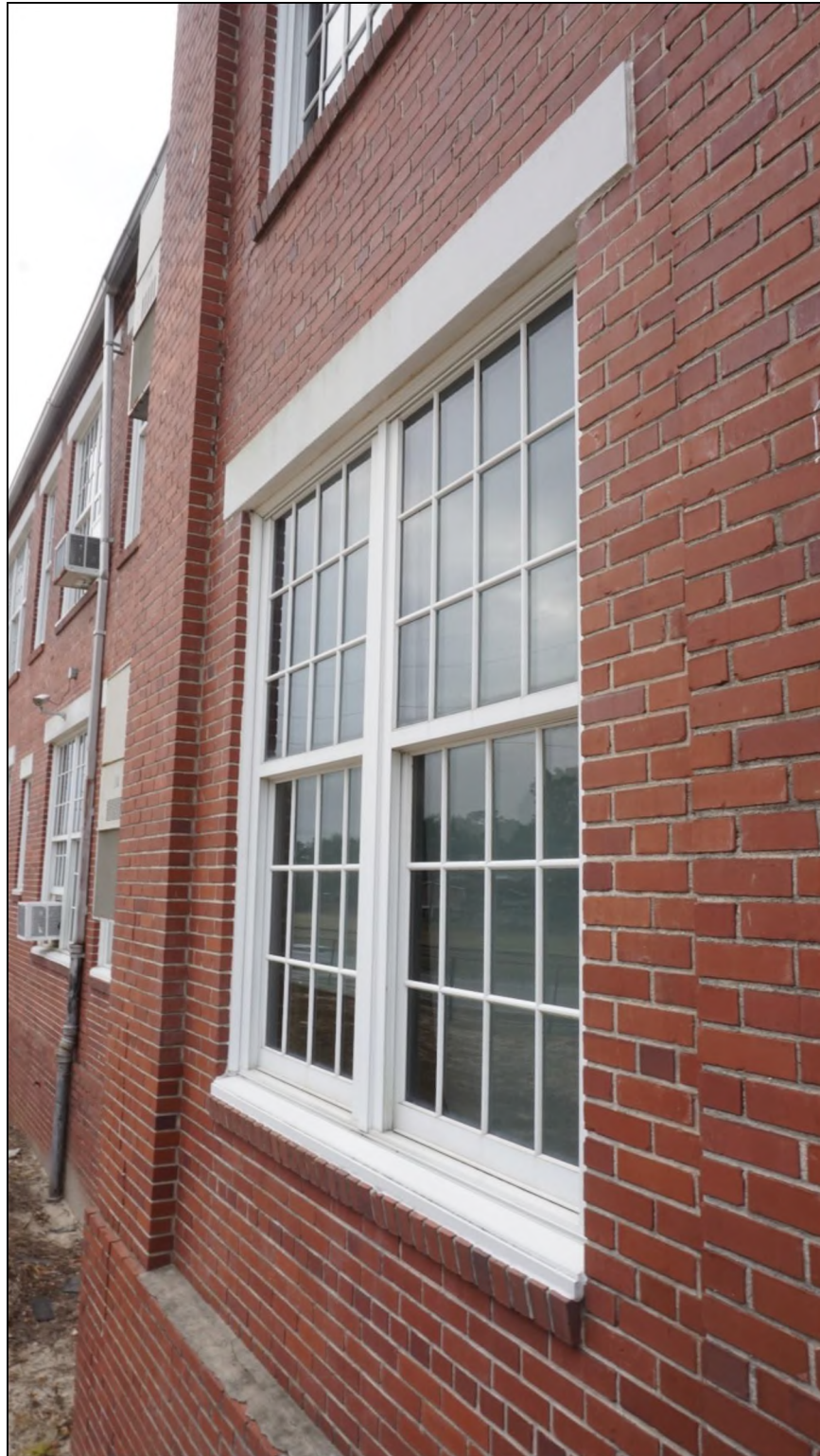
Figure 19. Twelve-over-twelve double hung sash windows located on the main structure.
