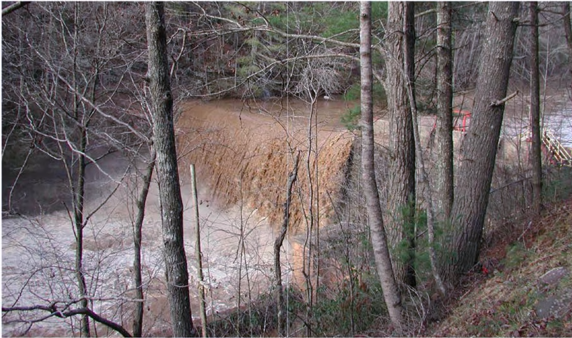
Photo 8: View of water leaving the project boundary, passing over the Woodside II Dam. Water contains an unusually heavy sediment load. Much of the sediment load is from upstream of Woodside I. It represents scour of residual sediment left in the river channel after dredging was terminated and erosion of the floodplain banks exposed after the dam was removed. Photo taken March 17, 2011.
