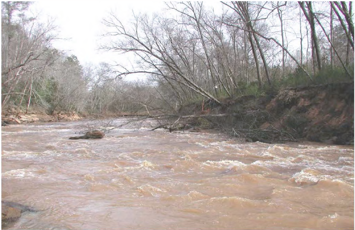
Photo 6: View of the river behind the former Woodside I Dam, after the dam has been removed. South floodplain (on the right) is collapsing during flow that followed a heavy rain (note trees have fallen into the river as banks collapsed). Photo taken March 17, 2011
