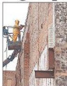
John Quenneville, an employee of DJM Enterprises, uses an air chisel to pry old bricks from the side of the building.
