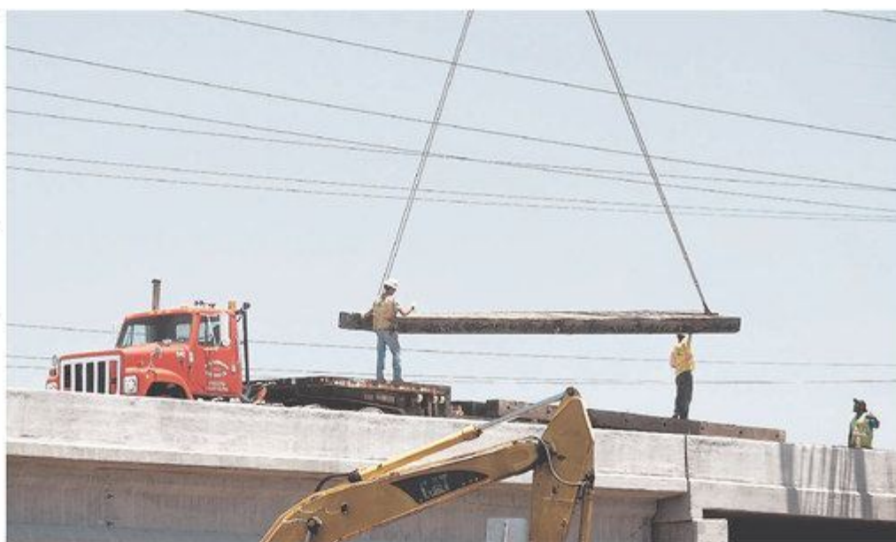
Workers with R. R. Dawson Bridge Co. help to guide crane mats, big pieces of wood that allow cranes and vehicles to drive on a marsh, onto a truck on Monday on the westbound ramp of the Bluffton Parkway flyover. The workers are cleaning up their equipment in preparation for the flyover to open.
