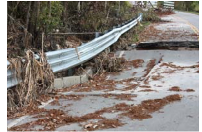
Bridge Damage at National Cemetery Road (S-13) in Florence County
