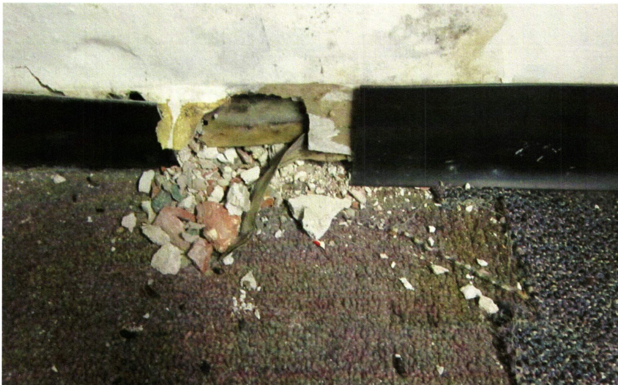
Rodent hole and rat droppings in the proposed museum space. Not also the mold and water damage to the wall board.
