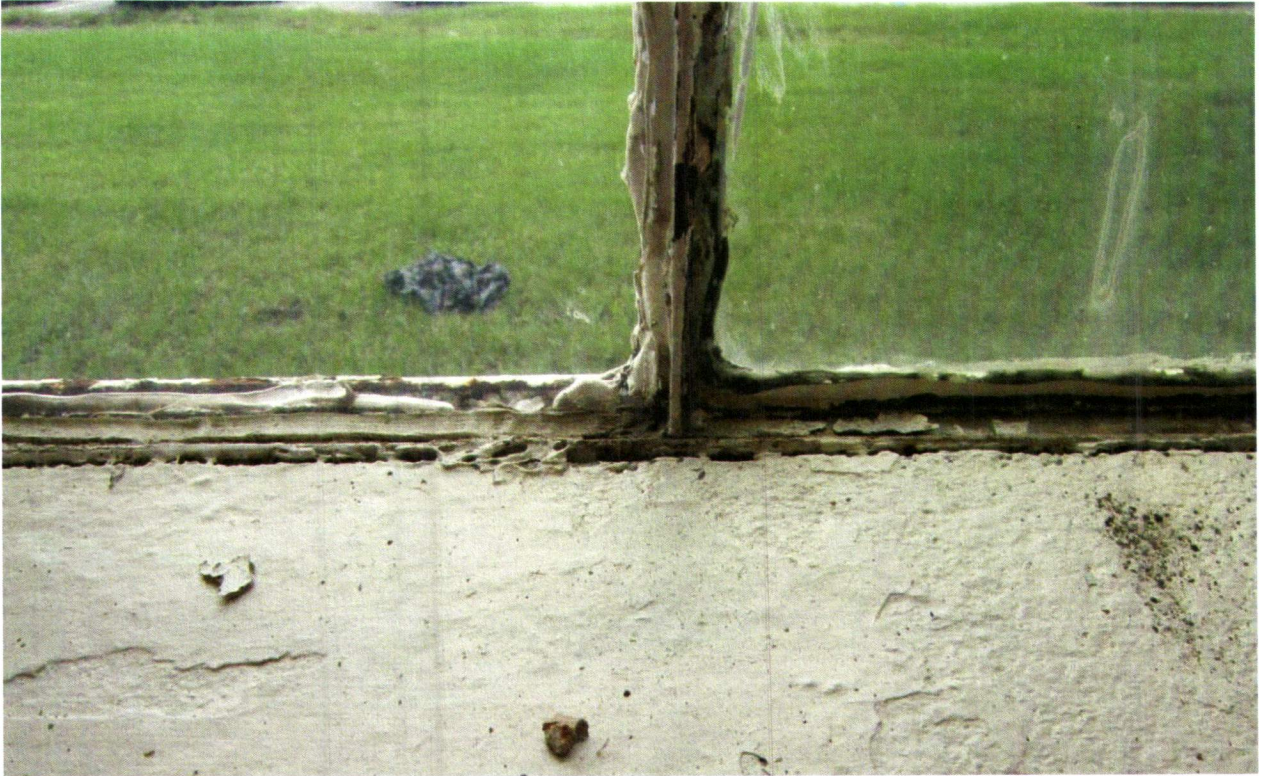
Close-up of metal windows showing deterioration and poor fit. They all exhibit a significant lack of maintenance and require extensive repairs.
