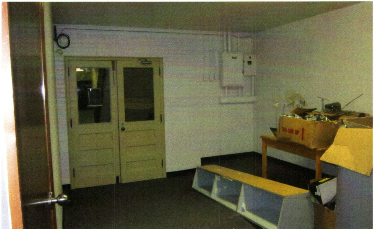
Double wood and glass entrance doors, not fire rated. They would need to be replaced. Electrical panel box to the right was locked and not available for inspection.
