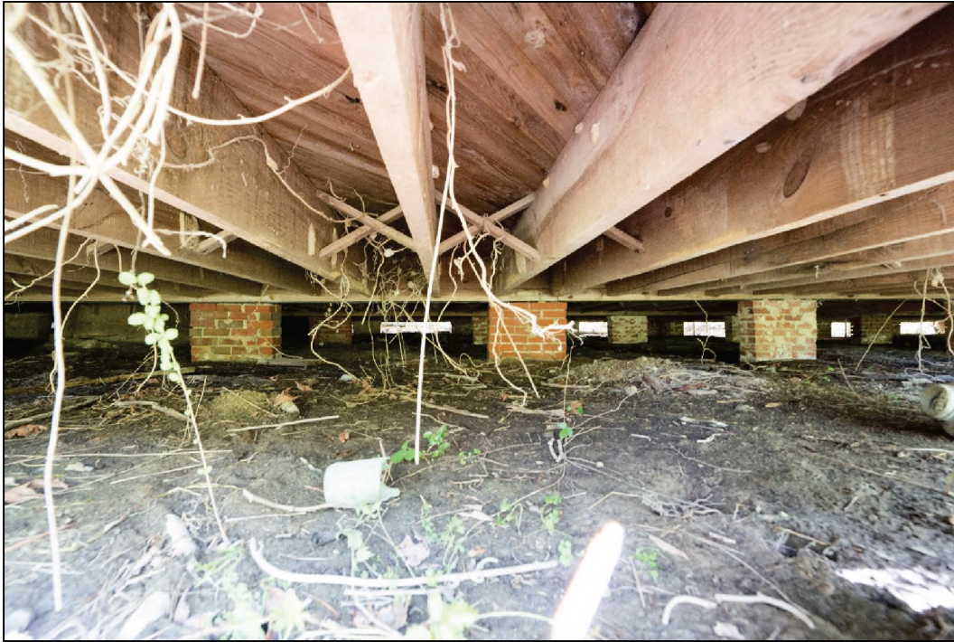
Figure 41. Brick pier foundation.
