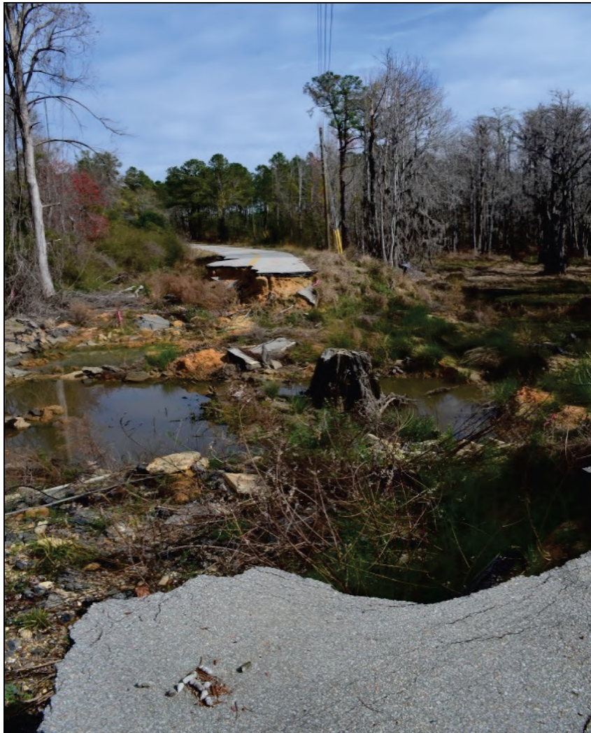
Figure 25. February 2017 view of the breach in the millpond dam/Old River Road, facing north.
