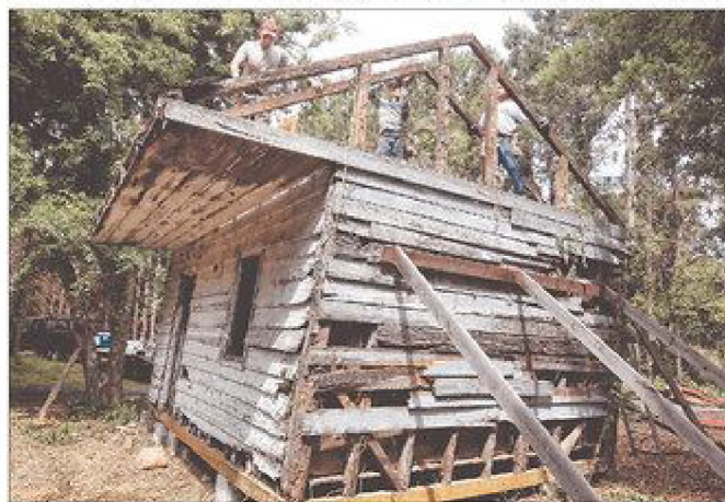
PHOTOS BY BRAD NETTLES/STAFF Ravi Munoz (from left), Ever Salamanca and Douglas Lundberg, with Museum Resources, remove the roof trusses from the Point of Palms slave cabin that is being taken down and moved to the Smithsonian in Washington, D.C.
