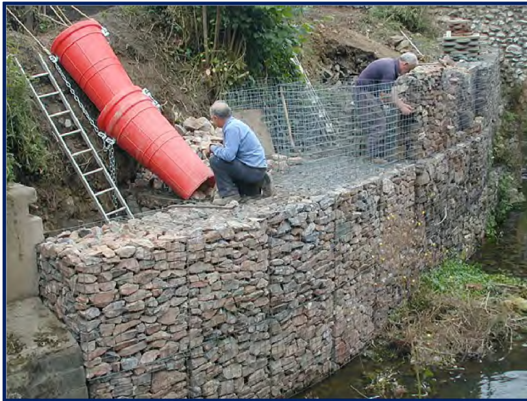
Installation of Gabions Similar to the Ones Used on Pheasant Branch Creek
