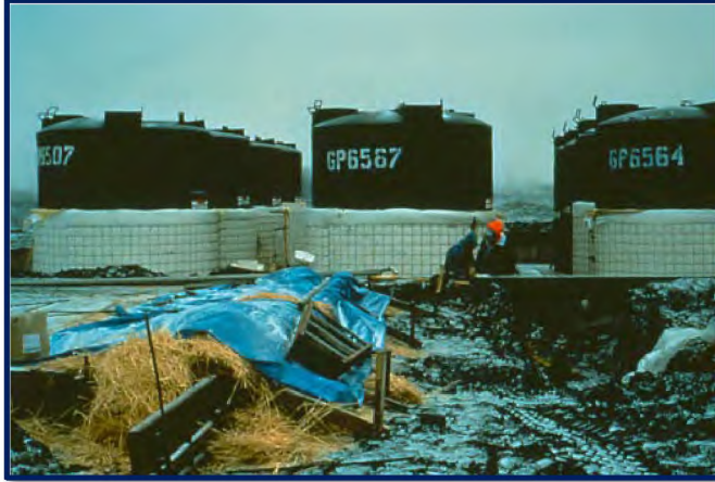
Temporary Tank Farm for Phosphoric Acid Used to Treat 350,000 Cubic Yards of Hazardous Melt Emission Control Sludge
