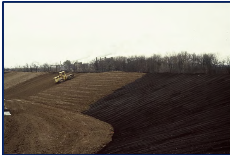
Clay Liner Construction with Industrial Secondary Material Core Berms
