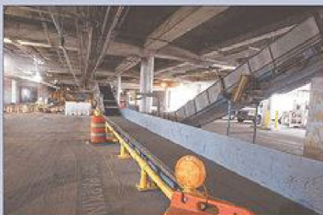
A new baggage belt has been installed in the underbelly of Charleston International Airport to support the third baggage carousel that was added.
