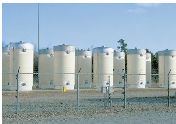
Fig. 1. (above) Wet storage of spent nuclear fuel in pools of water. When spent fuel is removed from the reactor it requires about five years in water to cool off and allow the short-lived radionuclides to decay away. It can then be transferred to dry cask storage (below) until needed, e.g., burned in Generation IV or V fast reactors in the near-future.
