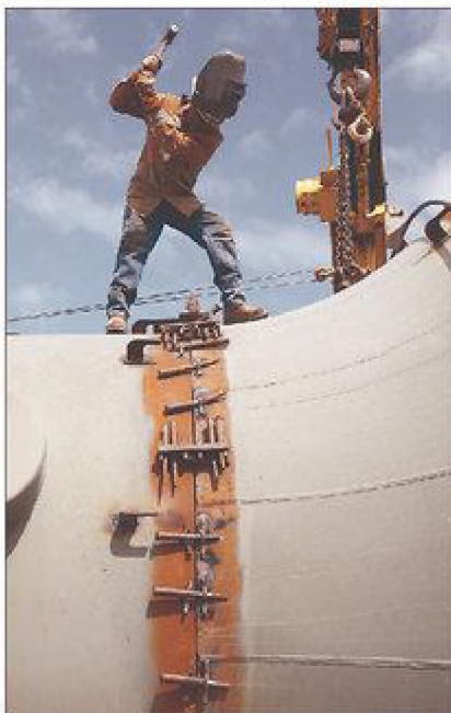
Salea Bor of Phoenix Fabricators and Erectors tightens steel sections of the riser shaft before welding it.
