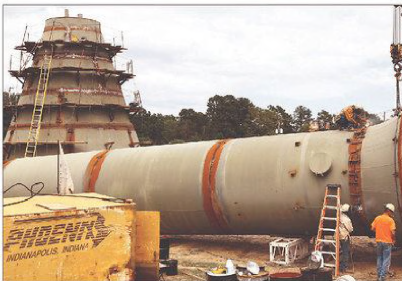
Salea Bor and John Arnold weld part of the new Pamplico water tower riser shaft along with Dan Zenner of Phoenix Fabricators and Erectors in Hyman on Aug. 25. Erection of the 200,000-gallon pedisphere water tower is expected to be complete by the end of September. At that point, paint crews will paint the base and shaft navy blue with a white tank.
