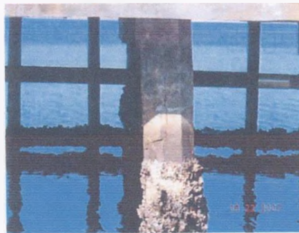
Figure 3: Pile with cracking near the cap.
