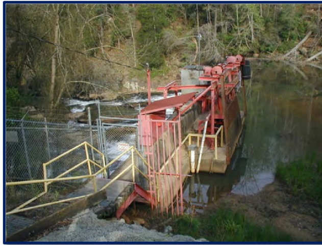
Sluice Gates and Penstock Structure Woodside I Dam
