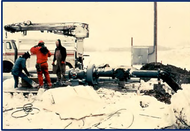
Installation of Blower for Landfill Gas Extraction System January, 1976
