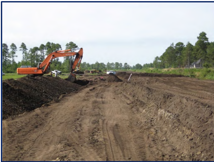
Land Development Earthwork after Clearance to Six Foot Depth
