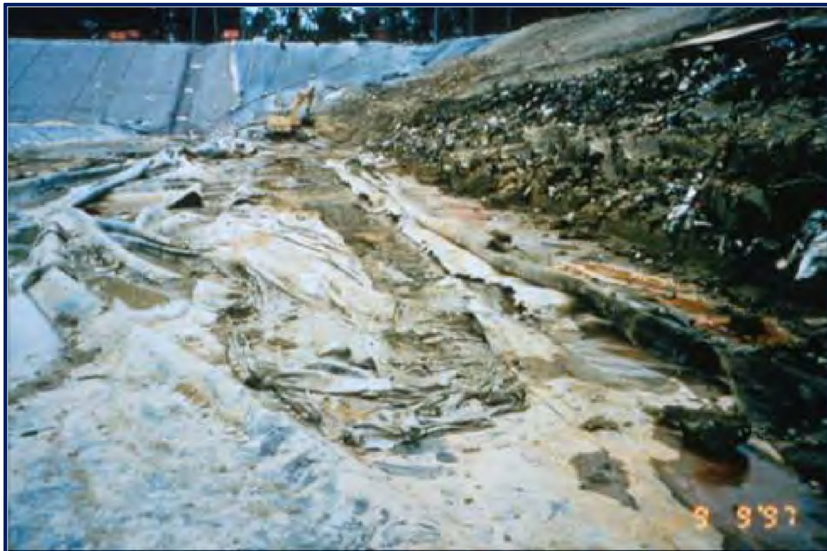
Intermediate Slope Failure Similar to the One between Cell IIF and IIG at Pinewood with damage to Newly-Completed Liner System
