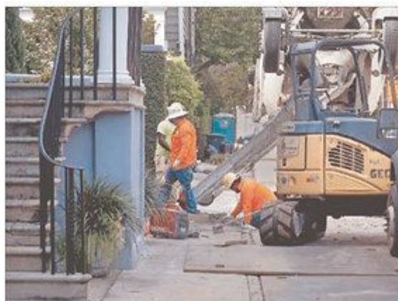
A crew from Gregory Electric Co. smooths out concrete Monday afternoon around new underground electric, cable and phone junction boxes on Orange Street. The overhead wiring is being taken down and installed underground after residents first requested it 17 years ago.
