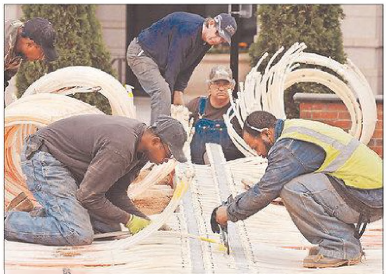
Workers, including Travis Syphert, left, and Jon Tubbs, right, put up cooling coils for the ice skating rink on Morgan Square in downtown Spartanburg on Tuesday afternoon. Skating on the Square will be returning for a fourth year; it is scheduled to open Nov. 25. TIM KINZEY/TIM.KINZEY@SHJ.COM
