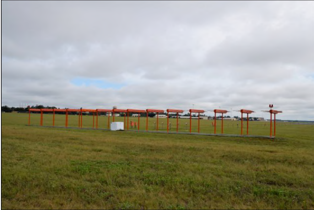
Figure 96. Facility 9172, ILS localizer array.
