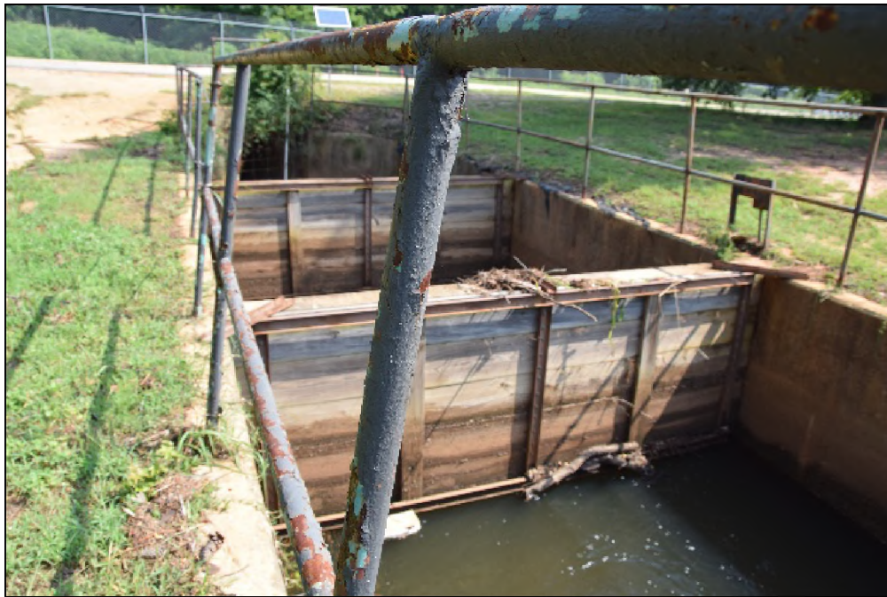
Figure 80. Sluice gate at Facility 9045.
