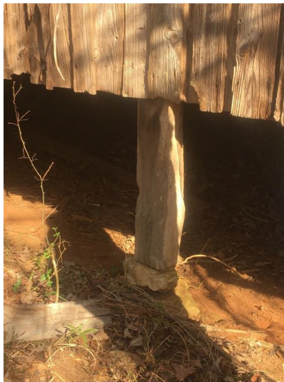
Photo 23. View of unstable foundation at northwest cabin (0278), looking north.
