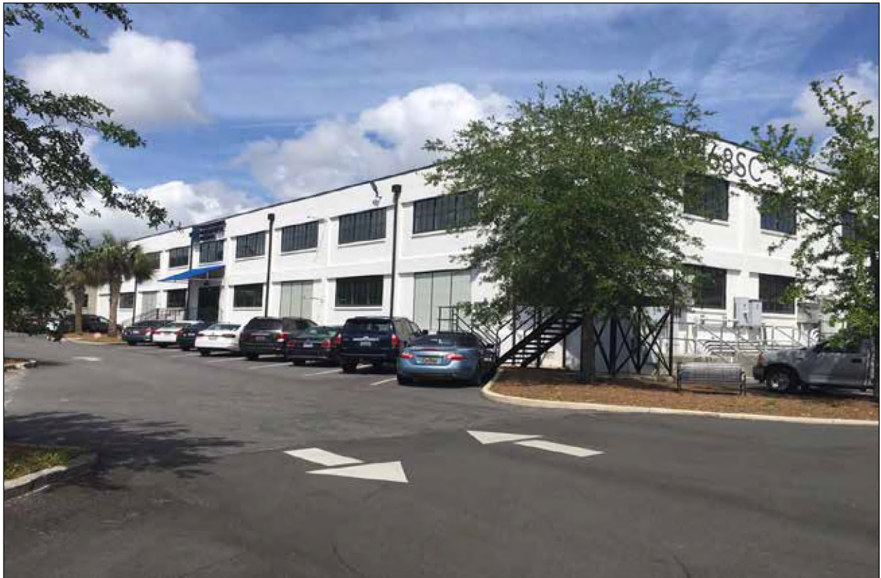
Figure 4.3 The Medical Supply Storehouse (NH68) at 1535 Hobby Street (looking northwest) has been rehabilitated and is in good repair but has replacement windows and bay doors.
