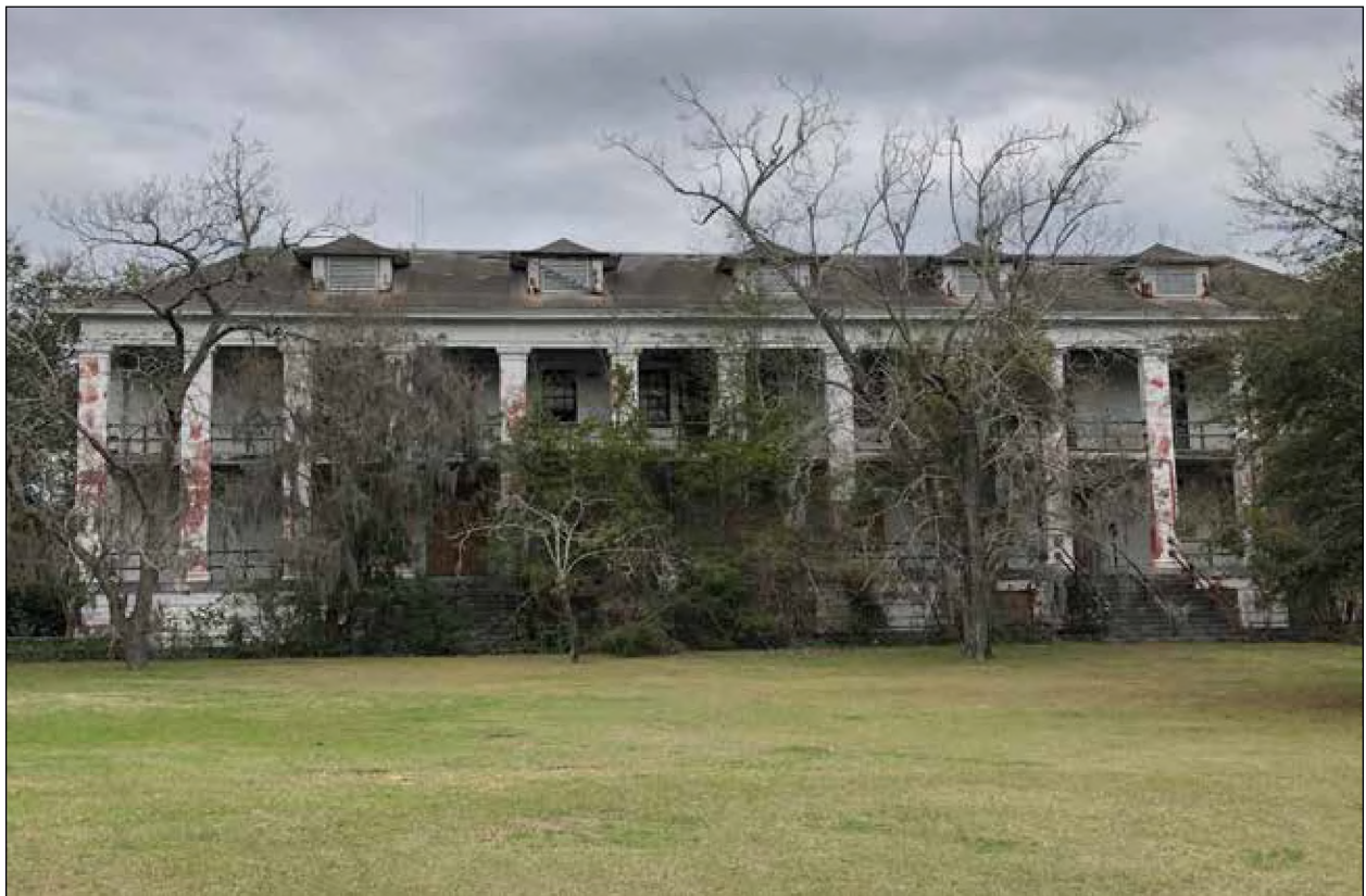
Figure 4.8 Marine Barracks Charleston (Building M-17, south façade, looking north) retains original architectural details and has had only minimal exterior alterations, but displays widespread disrepair due to water damage and neglect.
