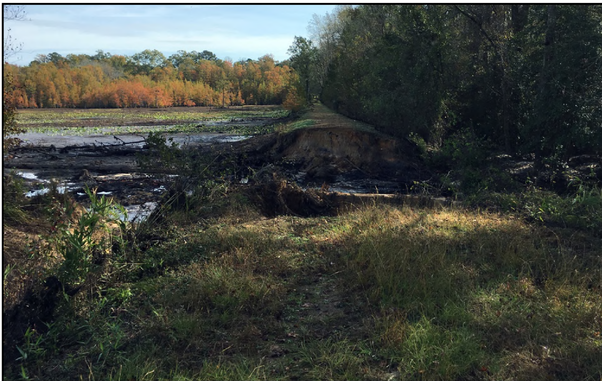
Figure 15. View of 2737.03 Showing Dam and Sluice Gate Breach, Facing East.
