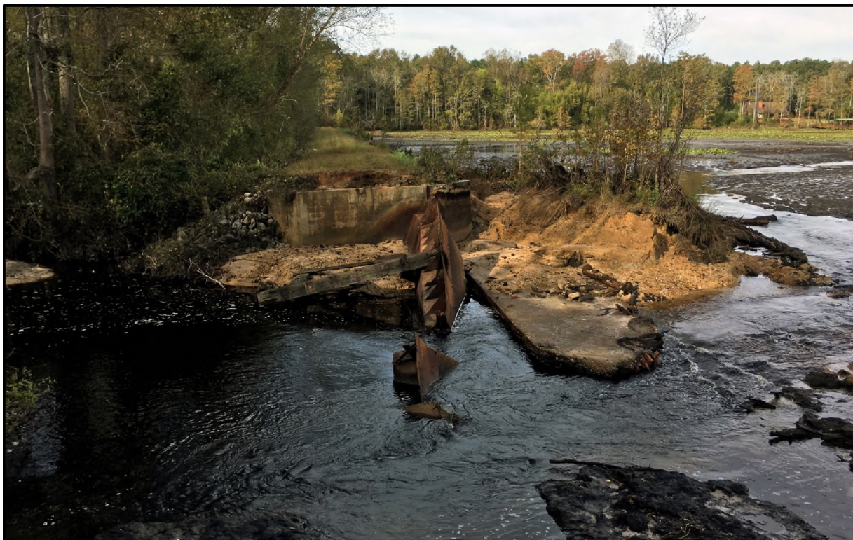
Figure 17. View of 2737.05 Showing Damaged Sluice Gate and Spillway, Facing West.
