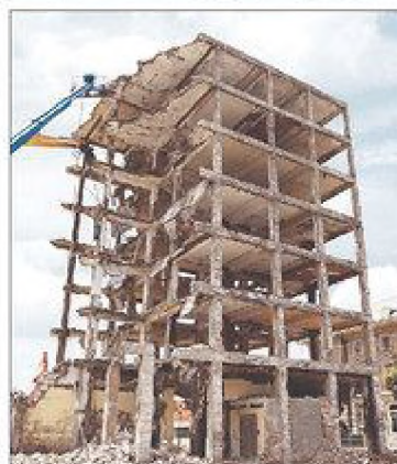
ABOVE: Wofford operates a 90-foot excavator to bring the concrete and steel structure down in a controlled manner. RIGHT: The Trust building on June 25.
