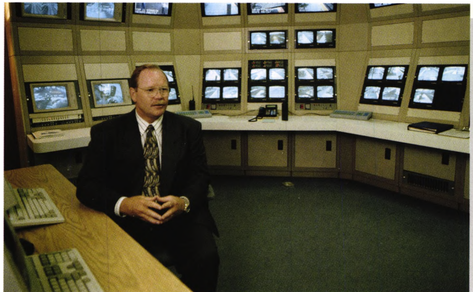
Security director, John Hanlon, shows off the central control room. For each station, small monochrome Cohu monitors display the signal from each camera, while a 19-inch color monitor can be selected for the color detail or simply a larger image.
