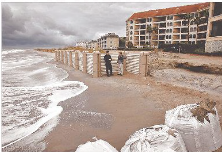
Deron Nettles (right), owner and designer of the wave-dissipation system, and Tim Mays, associate professor of civil engineering at The Citadel, say this new system will slow erosion much better than a solid wall or sandbags.
