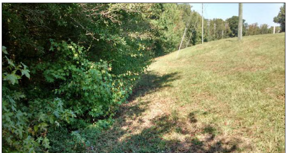
C. Most of the U.S. 521 Road Grade is Elevated Six to Ten Feet Above the Natural Ground Surface
