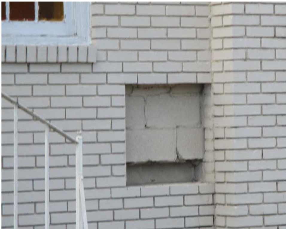
Figure 7. A section of brick removed from the church facade reveals a concrete block substructure (HDR 2017).
