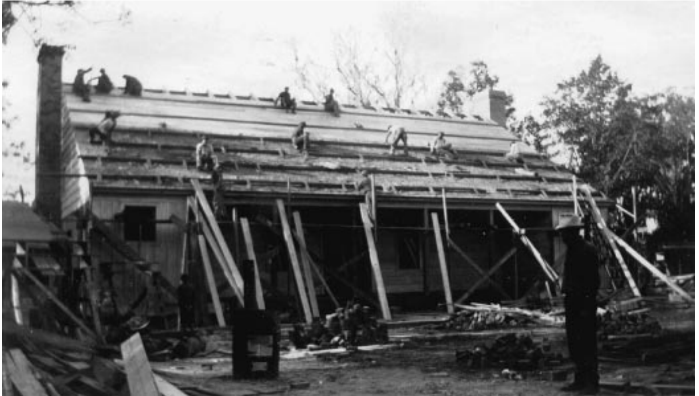
Roofing and shingling bath house.
