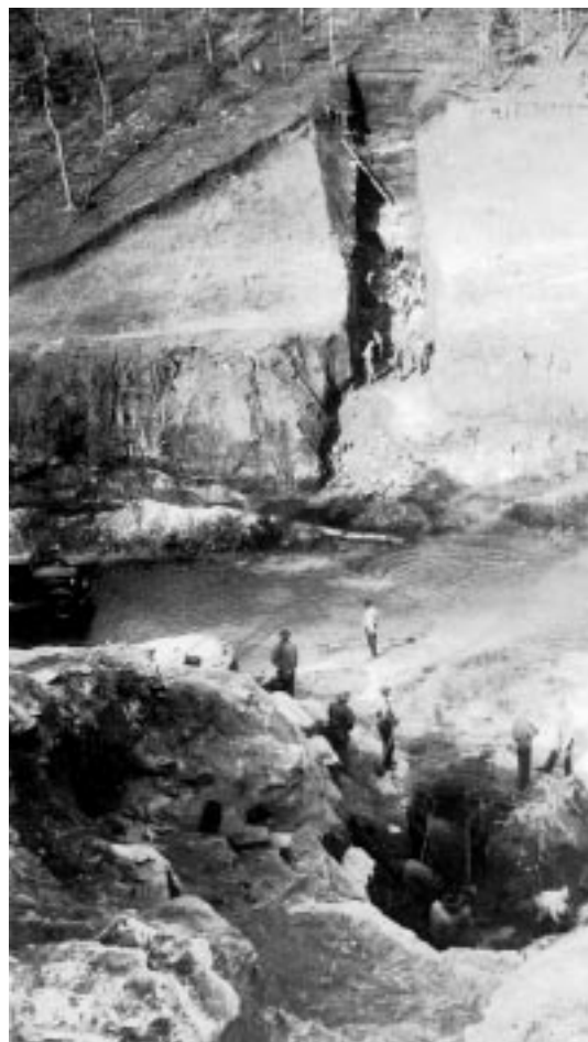
Core wall excavation.
