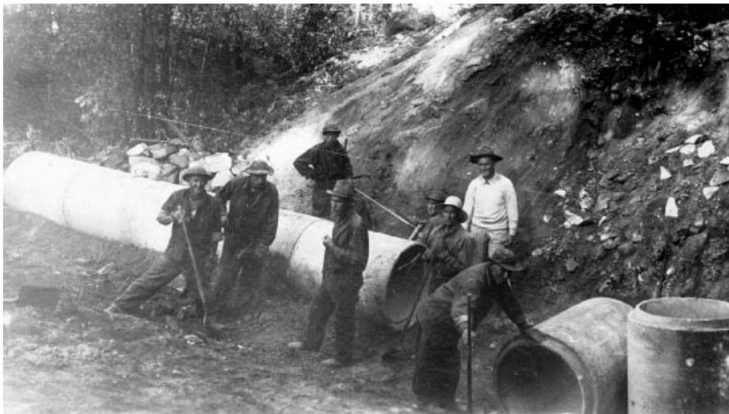
Laying concrete culvert on main road.
