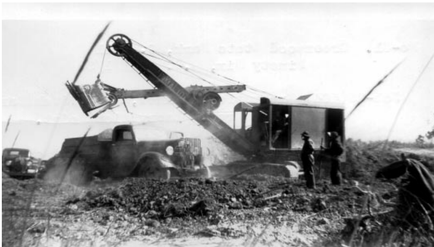
One yard gas shovel excavating channel/canal/ditch/Earth White Area. Observation Point.
