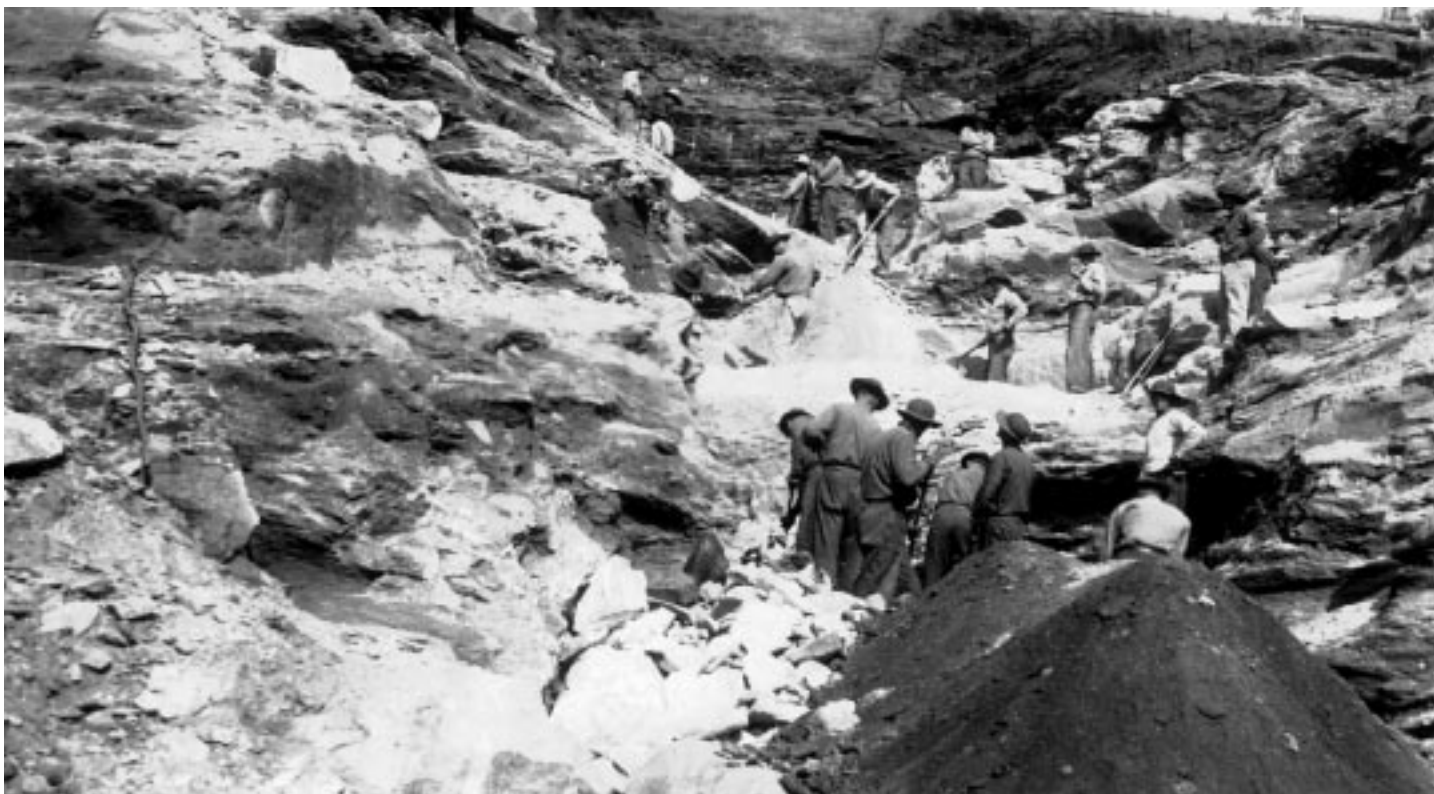
Rock excavation core walls dam site.
