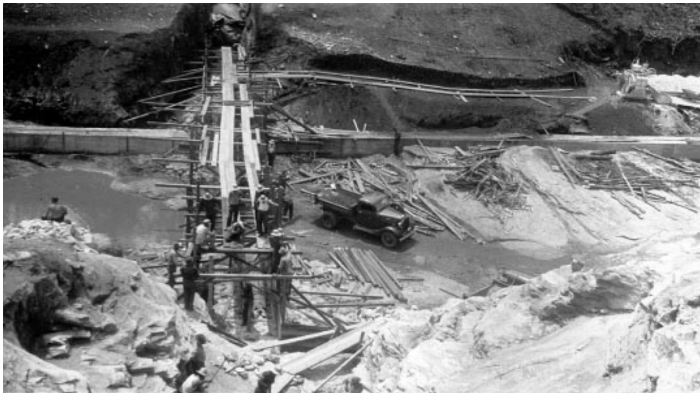
Building runways for pouring concrete in spillway section.
