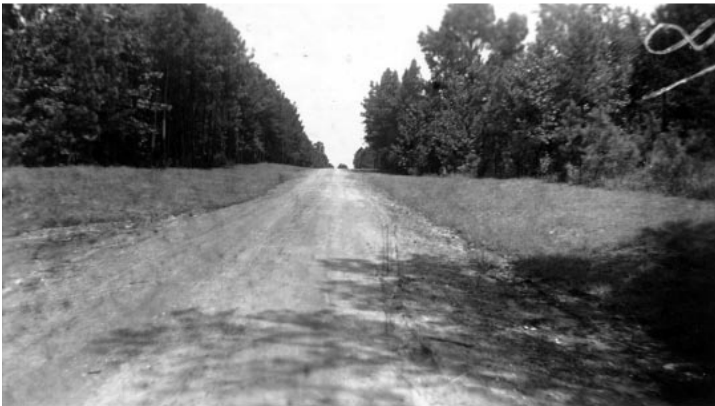
Road sloped (county road). Banks sloped and sodded with Bermuda grass.
