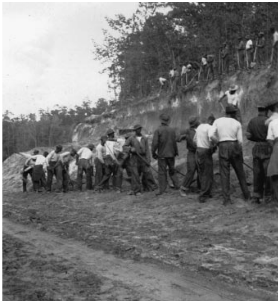
Excavating sand clay surfacing for park roads
