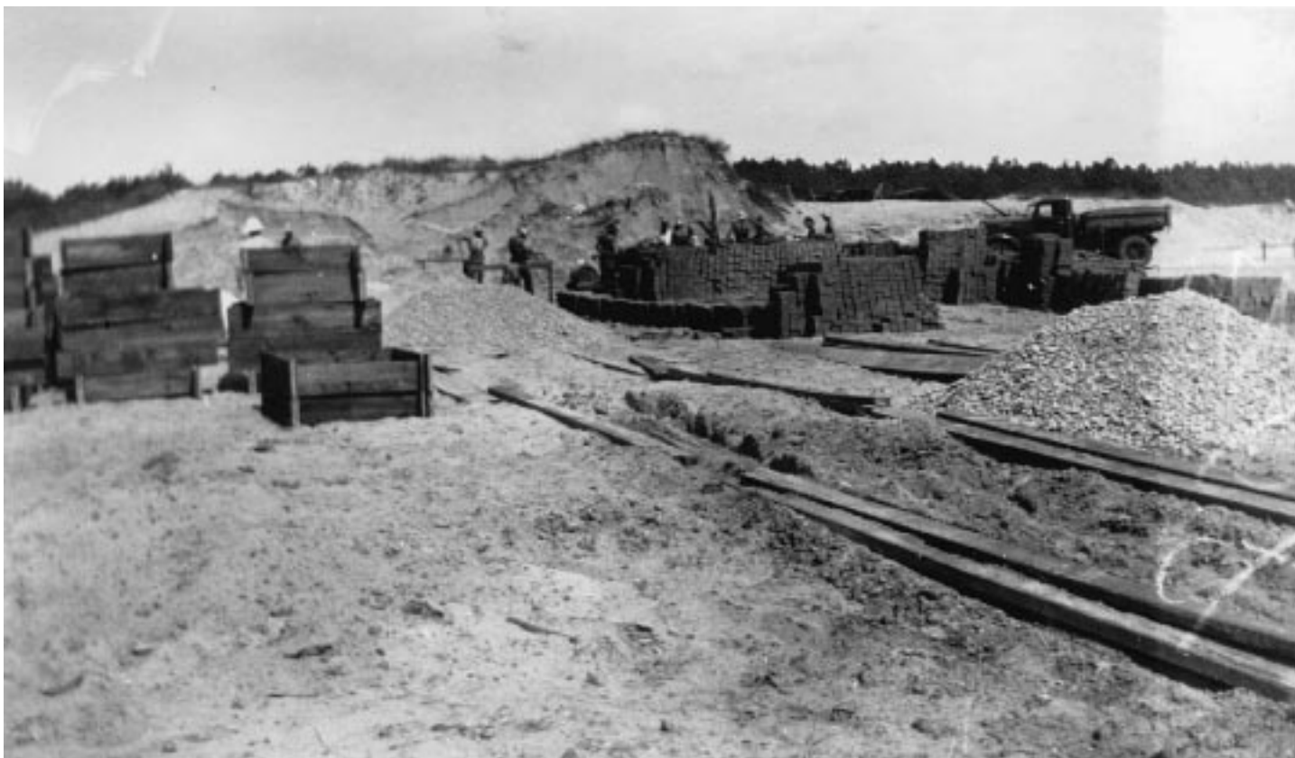
Brick, rock, and forms used in bathhouse piers.
