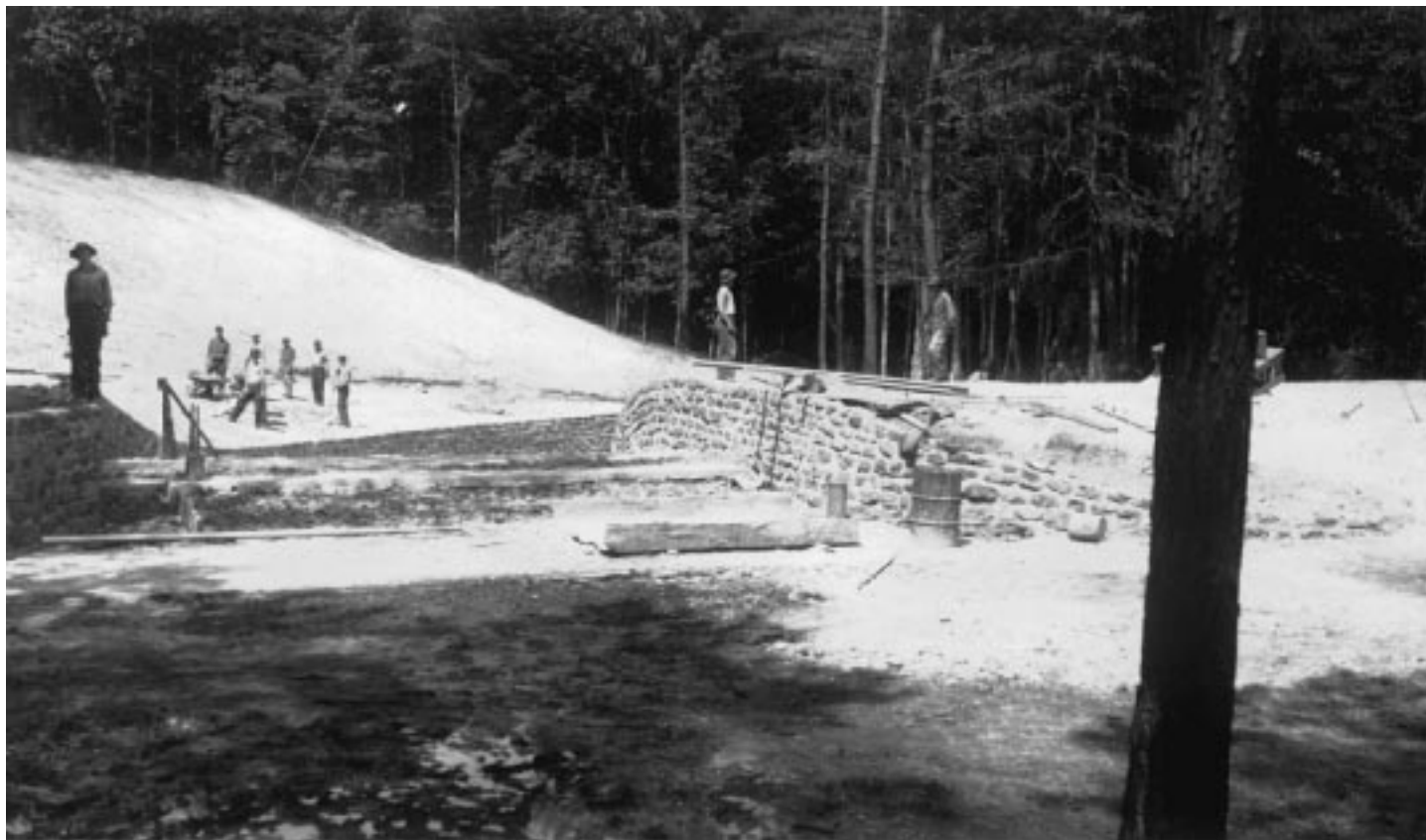
Rockwork complete on spillway.
