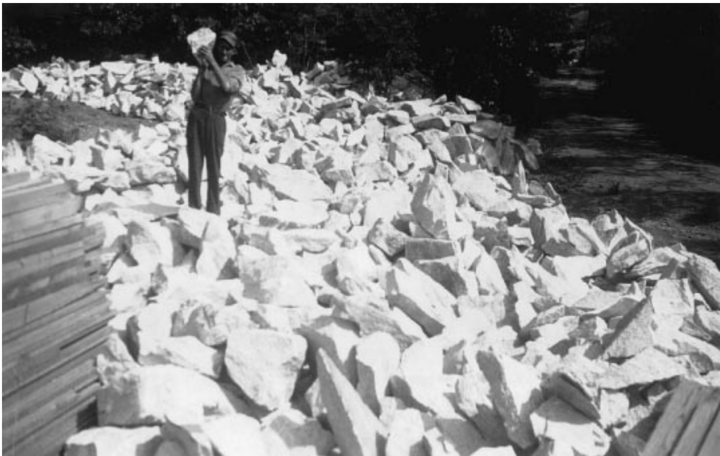
Stock pile of one-man stone to be used as plums in concrete work.
