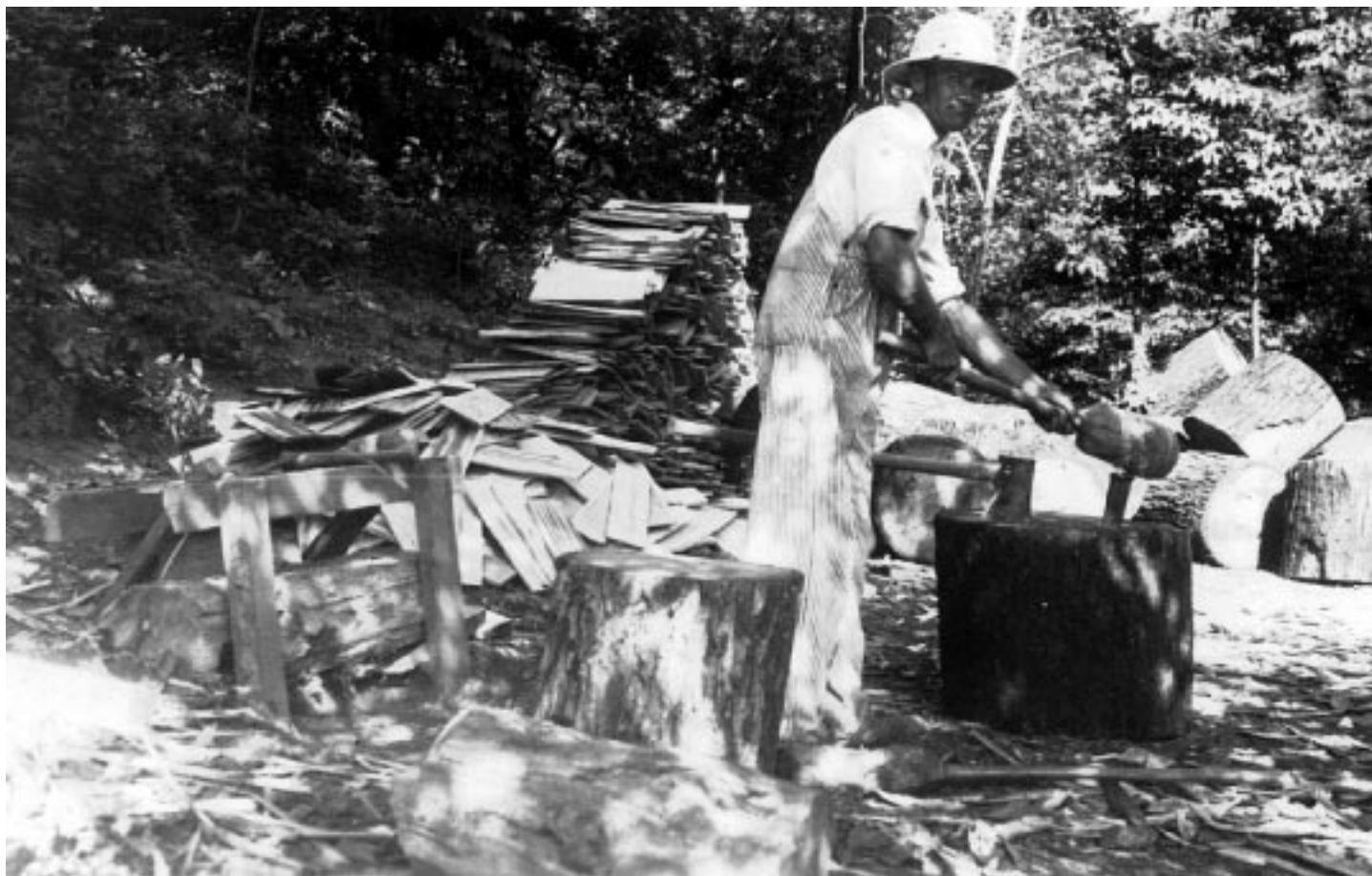
Making shakes for cabins.
