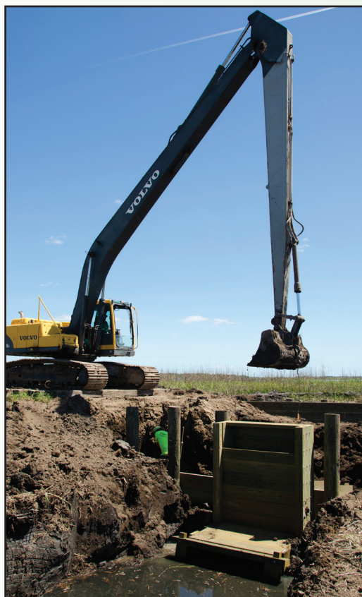
A new ricefield trunk was installed as part of the repair at Bear Island.
