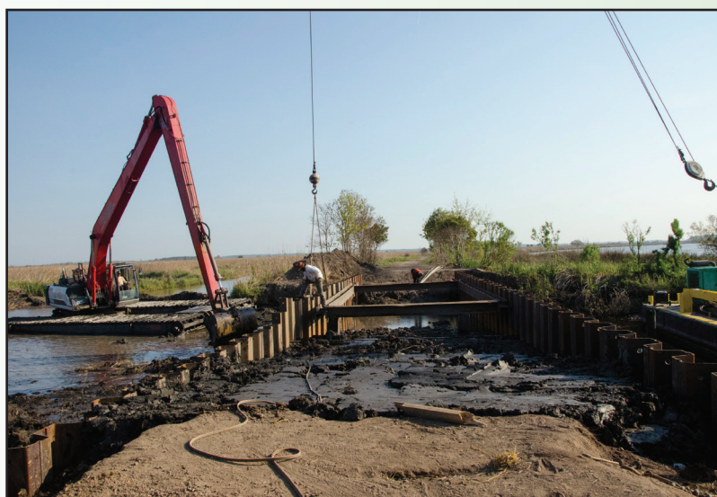
Workers install sheet piling to close a major breach at the SCDNR's Bear Island WMA.
