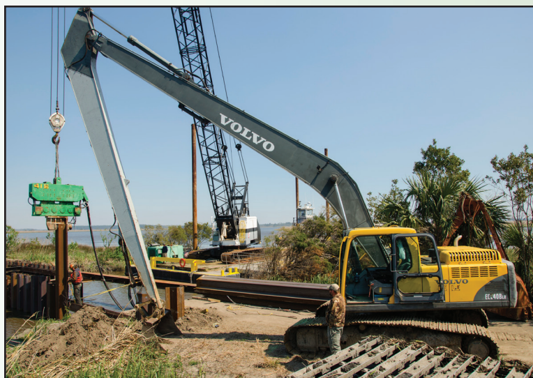
Bear Island wildlife biologist Daniel Barrineau watches as the crew from Wetlands Construction drives in a piece of steel sheet pile.
