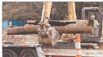
Crews on Wednesday removed a corroded pipe that caused a 500,000-gallon wastewater spill on Rifle Range Road.
