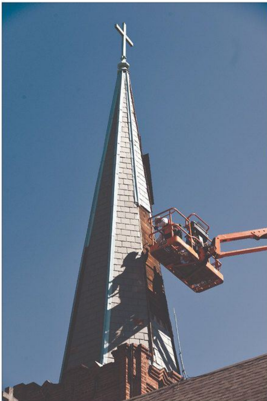
A Square-It-Up Roofing employee uses a hammer to pound in exposed nails on a steeple at St. Anne Catholic Church on Monday. The crew is replacing the slate tiles with typical asphalt shingles for the entire roof. The slate tiles had been on the edifice's twin steeples for 106 years.
