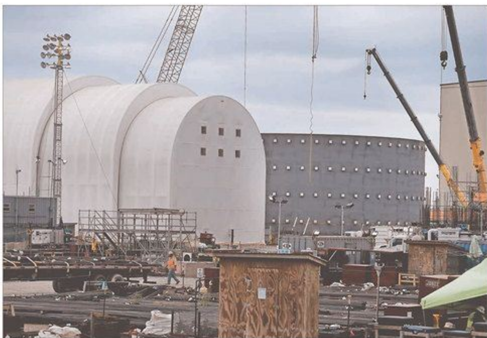
Rings were being constructed at the site of two new reactors at the V.C. Summer Nuclear Power Station in Jenkinsville in September. The rings were placed atop each other, creating the reactor.
