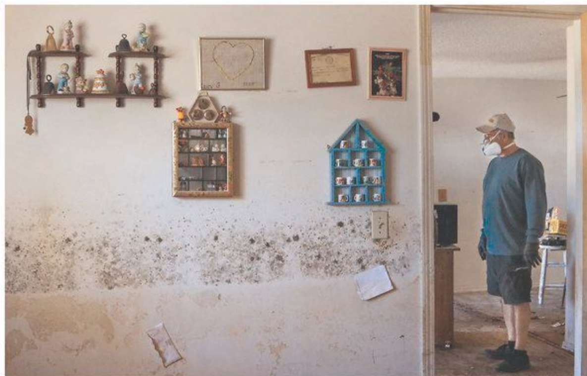
Dwight Dimery's Nichols home is covered in mold caused by flooding from Hurricane Matthew. The Little Pee Dee River engulfed essentially the entire town. Most residents suffered flooding inside their homes.
